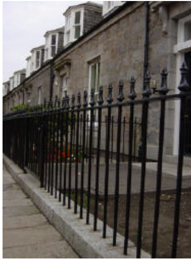
Railings installed to granite copes with lead
