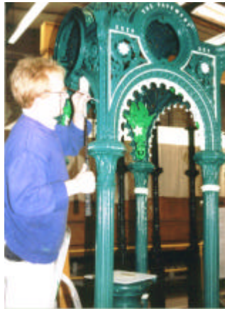
Canopy painted in workshop environment (Image courtesy of Heritage Engineering)
